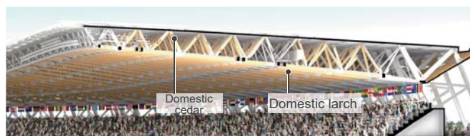
Image of using lumber for the truss of the Large Roof
