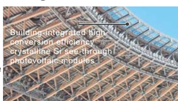
Image of photovoltaic facilities on the edge of the Large Roof
